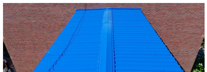
④ Roof of buildings and MH waterproof construction
