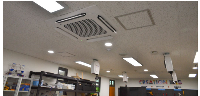
② VH 3rd floor Classrooms (G7-8 th homerooms) and other classrooms(ES Art room, Creation Lab) air conditioner replacement
