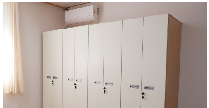
③ Dormitory air conditioner replacement and student's room furniture (single desk, bed mattress) purchase
